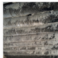
Before Dry Ice Blasting
