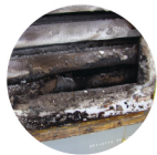
Before dry ice blasting
