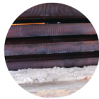
After dry ice blasting
